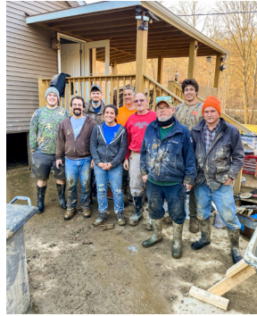
Work crew that helped Larry clean out the insulation.
